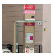
Small cells are playing an important role in the densification of Deutsche Telekom networks. Within the area that they cover, they provide a significant increase in data capacity; currently, up to an additional 150 Mbps. The new HUBER+SUHNER antenna range is enabling this increase in bandwidth using MIMO (Multiple Input Multiple Output) technology. Multiple antennas in a single housing allow multiple data streams to be sent and received simultaneously.
